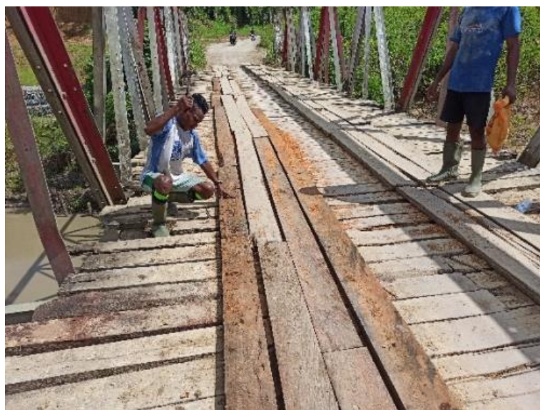
Figure 10. TAMI Bridge Maintenance
