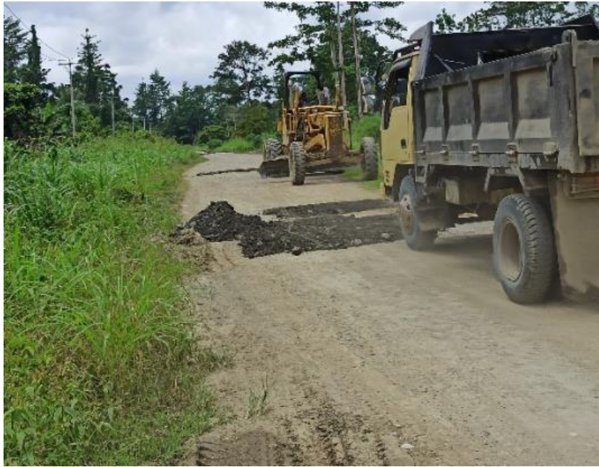
Figure 11. Road Maintenance in Yetti Village
